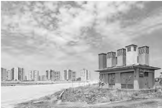
Figure 4. The new housing development is not constructed in a way compatible with the relatively harsh climatic conditions, which get very hot during the summers and cold in winters. The old Sur district has narrow streets, adjacent houses, thicker stone walls in older buildings and internal courtyards that provide comfortable living environments in all seasons. The new buildings are energy-inefficient and are devoid of regional character since they look the same as buildings anywhere else in Turkey. ©Murat Germen, 2016.
