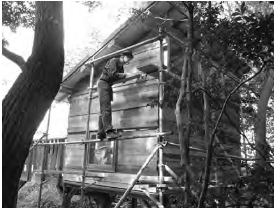
Figure 16. Making the walls of the house (2010)
