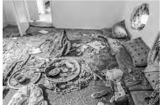
Figure 9. This was the saddest moment I personally experienced, which was surely not sadder and more brutal than what some civilian residents of Sur district suffered; loss of homes, injuries, even death... The large hole on the wall in the right-hand side is a puncture caused by a loose artillery shell, that instantly killed an old woman having a meal at her home, away from the conflict area. The place was left as was and nobody has cleared the scene, including the relatives of the old woman. ©Murat Germen, 2016.
