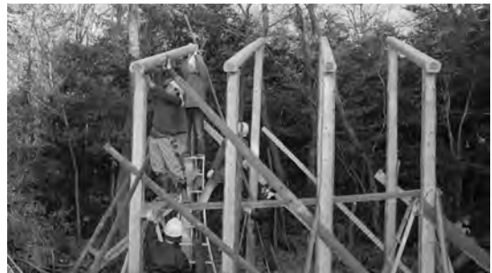
Figure 15. Raising the house beams (2008)
