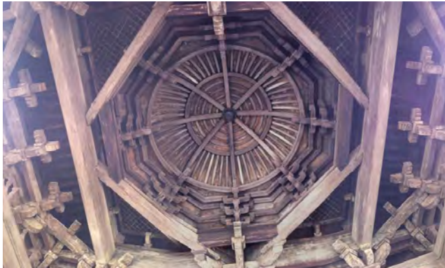
Fig. 4. Jinci temple, Shanxi province, built 1023-1032 CE, Song Dynasty corbels and post and lintel roof structure. Image, Hursty.
